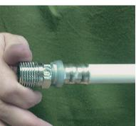
The press procedure has been completed.
