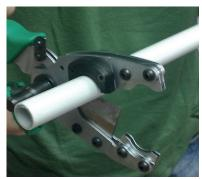
With the use of the appropriate cutting tool, cut the pipe vertical attending not to be warped.
